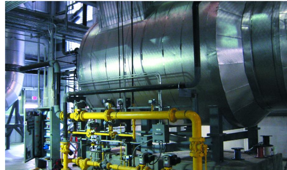
State-of-the-art hot gas generators (HGG) for any process requiring a heated air stream.
