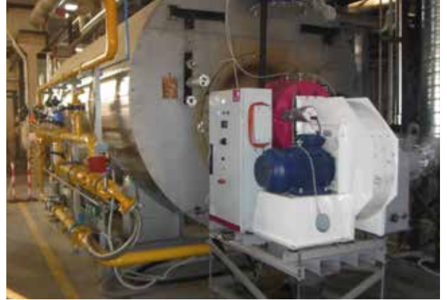
Pillard NANOxFLAM ® already implemented in more than 100 boilers (fire, tubes, water tubes)
