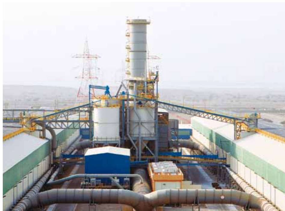
Sohar Aluminium Gas Treatment Center
